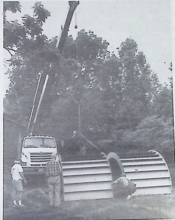
Crews prepare to place the two sections of water wheel at Mapleton Mill. The wheel was restored in Dayton and transported to the site near Churchville.
